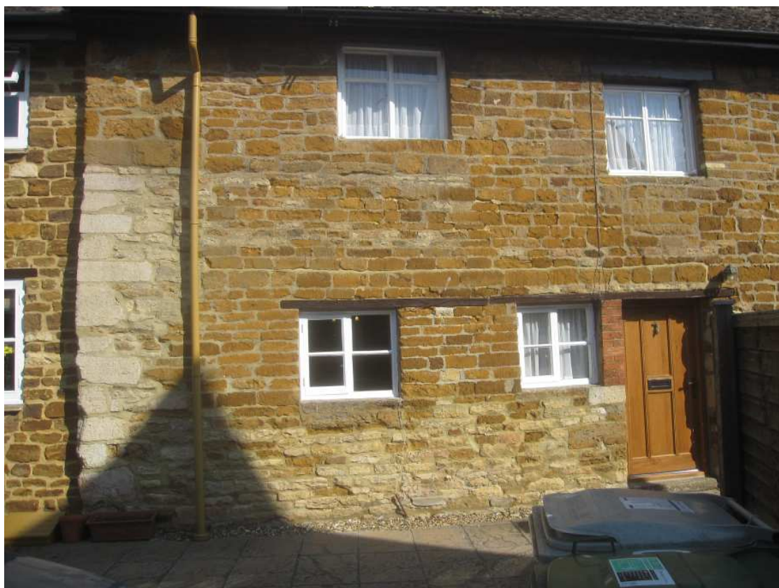
The south side, with original limestone quoins to left
